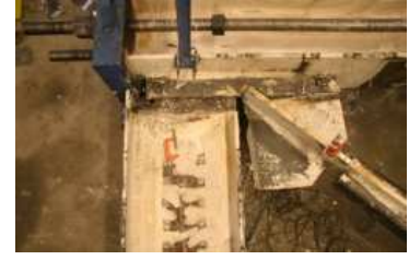
(c) Weld failure of gusset plate[7]
